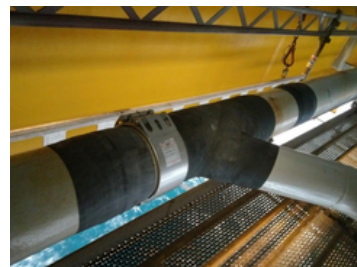
8" Open Drain Wrapping Offshore
